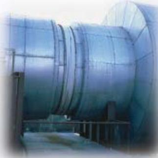
There is no more demanding service for expansion joints than wet scrubbers. Senior Flexonics Pathway can provide the correct PTFE or FKM gas seal materials to handle this hostile environment.
