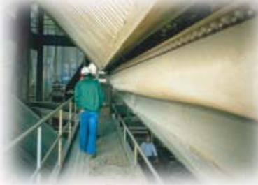
Our fabric expansion joints are ideally suited for this flyash laden application. Flexible high strength and lightweight fabric belt elements in
