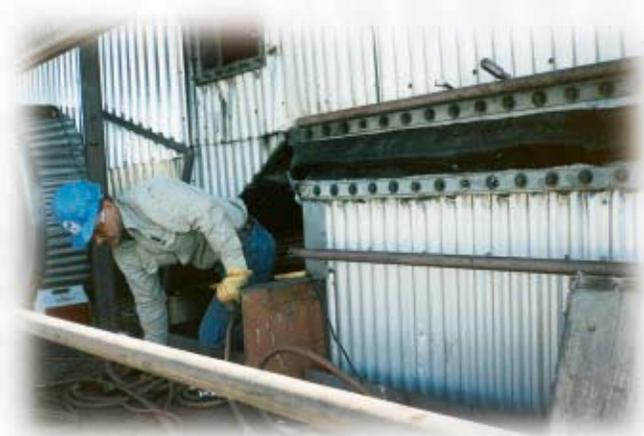
Field survey technicians perform comprehensive inspection of all expansion joints and provide a written and photograph document to plan replacement based on existing and projected life expectancy. Infrared analysis determines leaks even if the expansion joints are lagged over. This methodical approach reduces/eliminates the potential of unplanned forced outages and accurately projects the scope and cost of outage work required.
